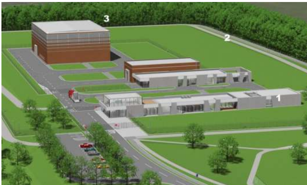
Figure 5-3 Display of spatial placement of individual repository facilities: 1 Administration and service facility, 2 Technological facility, 3 Hall above silo [18].
